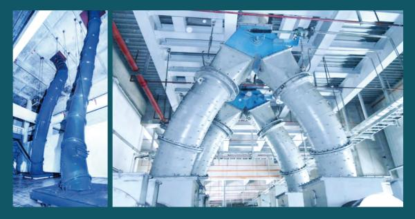
Our custom chute lining protects the chute from the material being handled. Skirt Liners prevent fugitive materials from escaping and damaging the conveyor loading areas. By combining the right liner with the correct chute design, we improve overall system efficiency and maximize material transfer, promoting efficient flow, dust suppression, and reduced buildup inside the chute.
